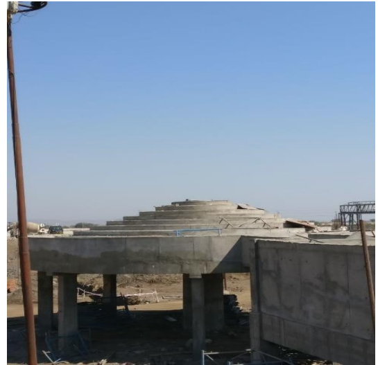
Fig 2.6: Cascade Aerator
